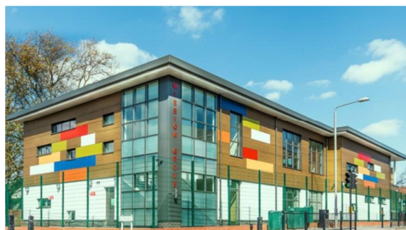
An example of the innovative modular construction
